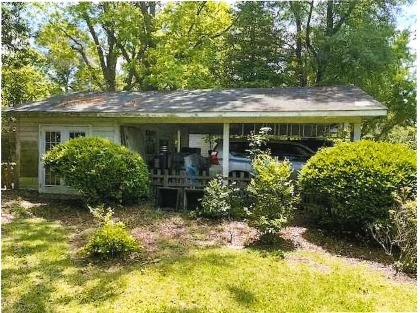
5 5-Left OV Left elevation; from backyard
